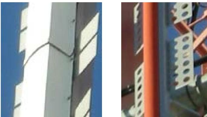
Typical plastic strip slot covers of competitors side mount UHF slot antennas. The square shaped white one is more prone to ice build up.
